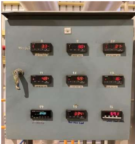
Temperature Monitor panel (Bearing, Oil lube, Steam)
