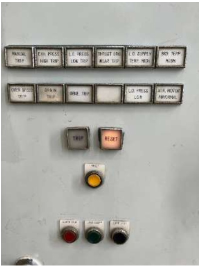
Turbine starting panel
