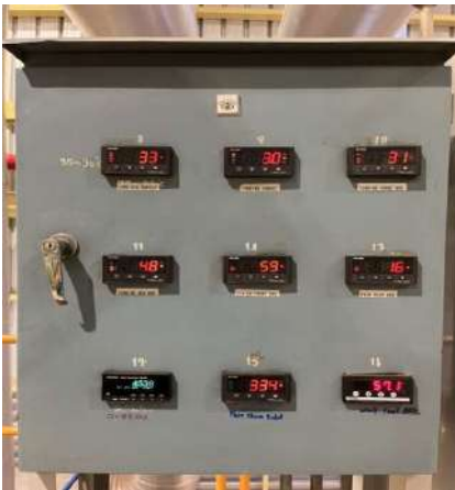
Temperature Monitor panel (Bearing, Oil lube, Steam)
